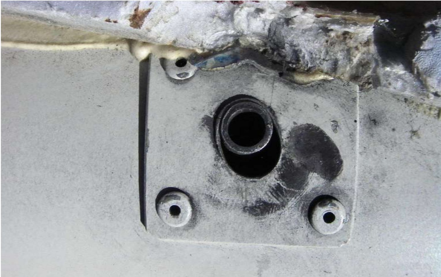
Photo 6 Port side of boom at rear hanger attachment, showing at least 4.5mm ovalised wear (in 2mm thick port backing plate)
