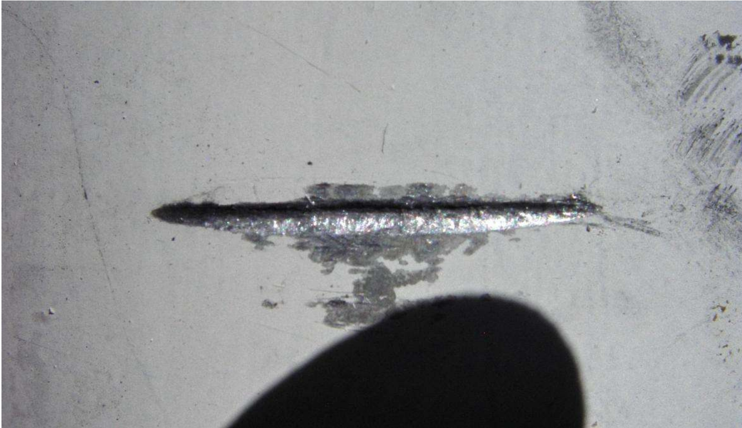
Photo 2 Groove across underside of boom (25mm long x 0.6mm deep) worn by the rear hanger gusset
