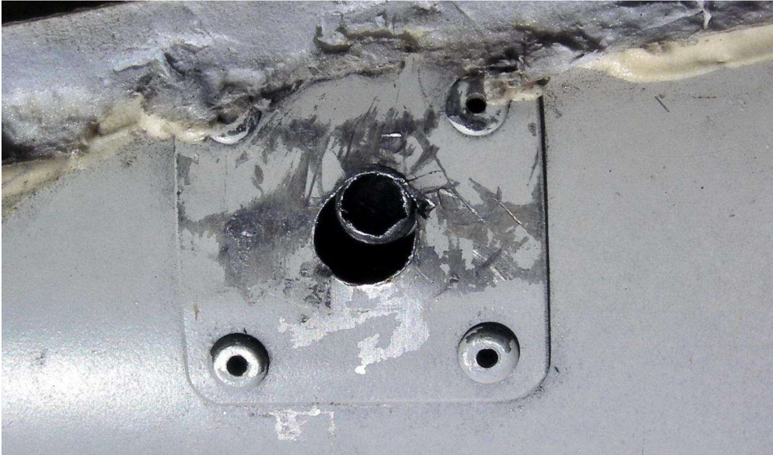
Photo 5 Starboard side of boom at rear hanger attachment, showing at least 5.0mm ovalised wear (note under-length alloy spacer tube and 1mm thick backing plate)
